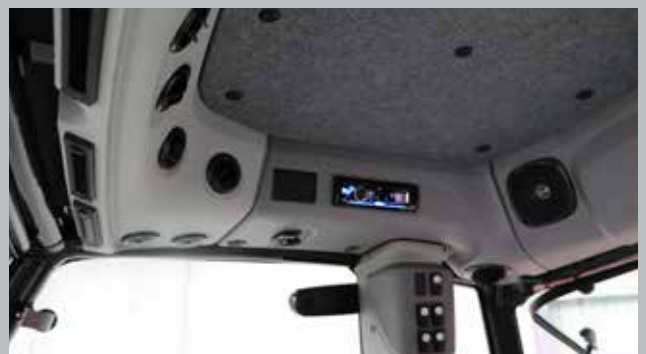
Air vents located throughout cabin.
